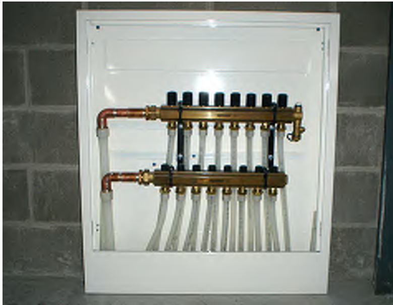
Radiant manifold in a wall cabinet (sample)
